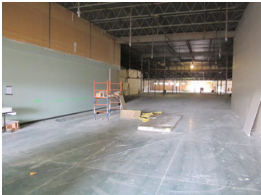
Renovations have begun to transform the former mall once again.
