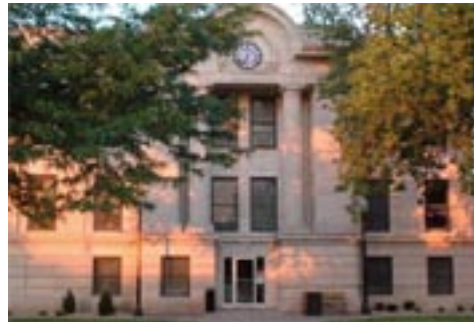
Phillips County Courthouse
