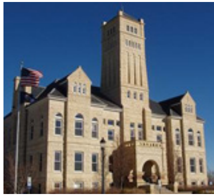
Geary County Courthouse
